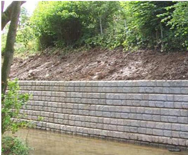
Figure 2.3 – Blockwork wall with embankment
