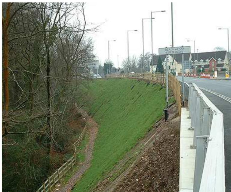
Figure 2.1 – Stabilised slope with topsoil retention
