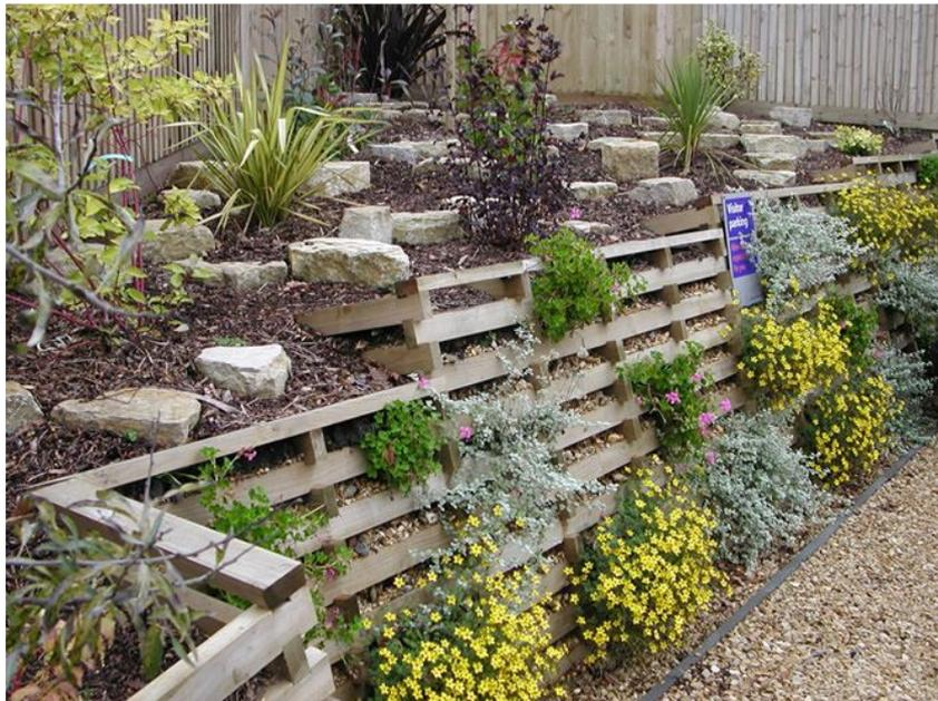
Figure 2.2 – Timber crib wall with planting
